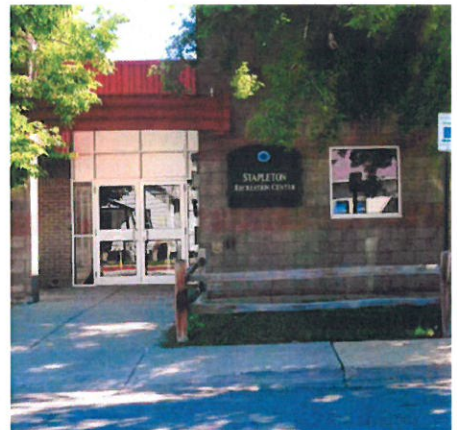
Stapleton Recreation Center
